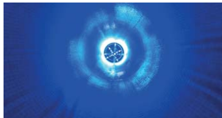
Neuer Bluelight PAA-GF-Liner DN 500 mm
